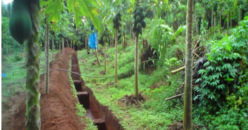
Lock and Spill drain on cultivated land (Source: SriCAT)
