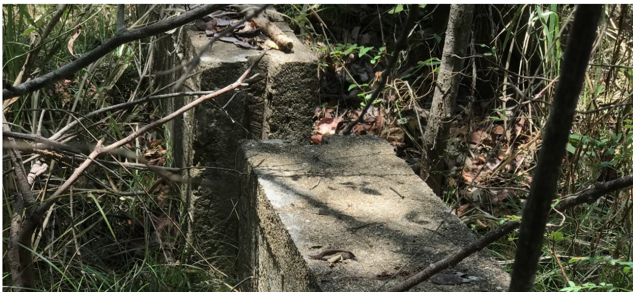
An abandoned sluice gate
