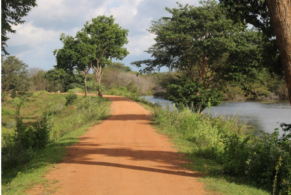
Figure 8: Repaired bund of Thumbikulama Tank
