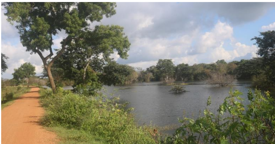
Figure 5: Site view of Thumbikulama Tank after restoration (2024)
