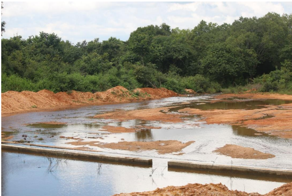
Figure 9: Repaired spillway of Thumbikulama Tank. (The spilled water runs to Bellankadawala Tank)
