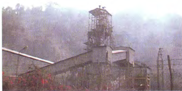
Photo 10.2 Fugitive emissions at a limekiln unit
