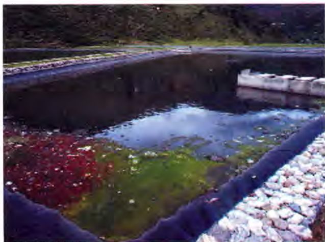
Photo 11.5 Sewage treatment plant
