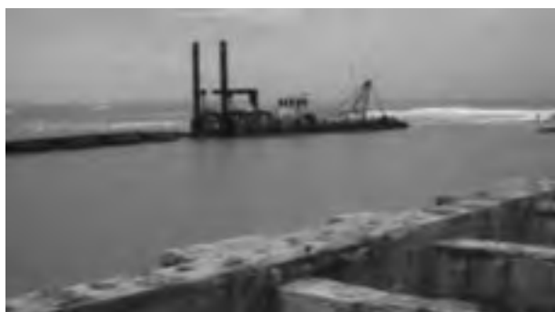
Figure 6. Dredging operations at Ennore Creek, Chennai to remove accreted sediments
