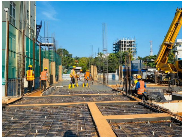
Ground-floor form and reinforcement work
