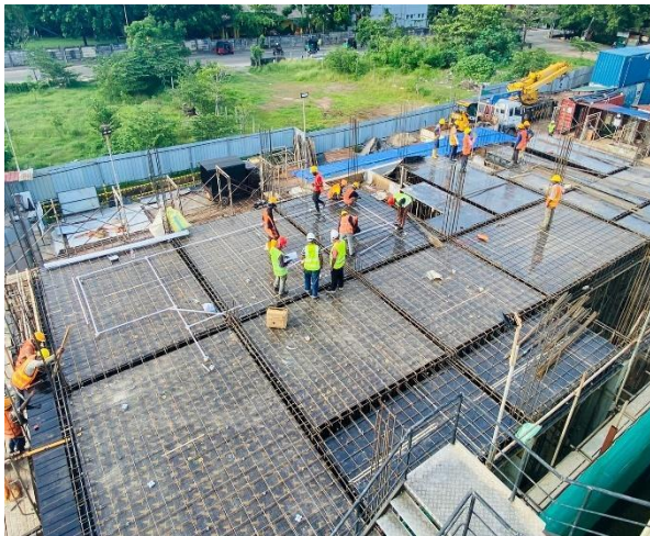
Ground-floor form and reinforcement work
