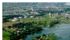
Oil leak from Petrotrin's fuel tank reported at Point-A-Pierre
